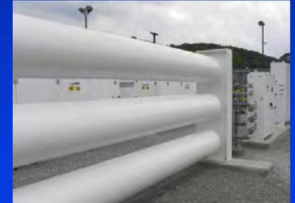
...or compressed and distributed directly to vehicles' onboard storage cylinders (time-fill applications)
